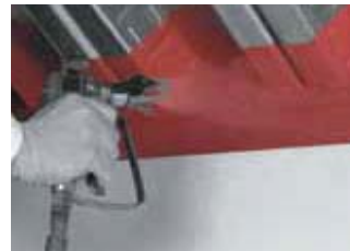
Superior finish smooth surface allows quick and cost effective coverage with Hilti CFS-SP WB Firestop Joint Spray.
